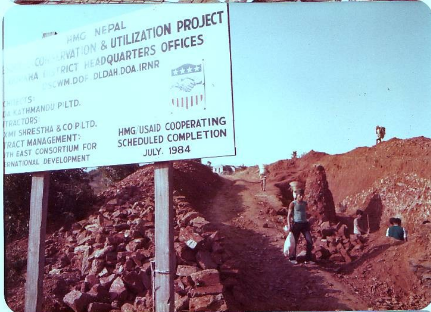
road works at Gorkha, siang was responsible for design of this road
