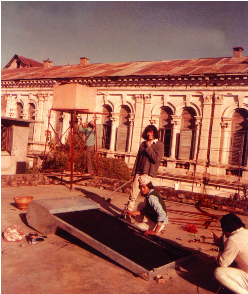
Kathmandu Nepal 1982 Siang installing the first multivavle solar heater in the world on the roof of his house at Hitti Durbar, Kathmandu.
