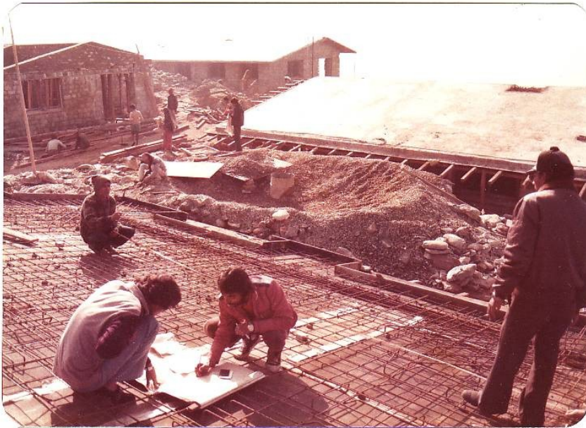
Construction works in progress at RCUP Headquarters Com- plex, Gorkha Nepal Feb 1984.
