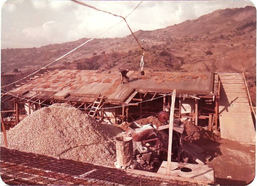
note "cut outs" in eaves above south facing bedroom windows in this Type A officer's quarters for passive solar gain in winter
