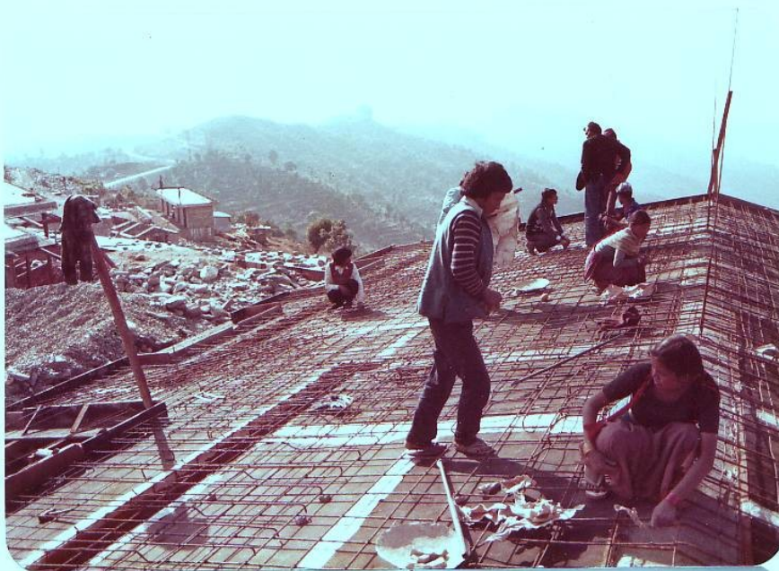
checking reinforcement of roof slab
